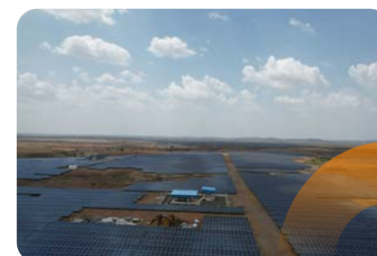
SuryaCon - Best Performing Project of the year-100 MW and Above (Dhule 150 MWp)
