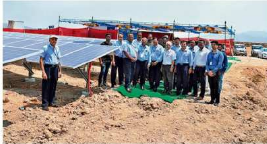
The solar panels installed at the Tirupati airport complex at Renigunta.
